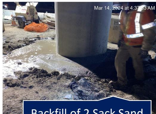
Backfill of 2 Sack Sand Slurry for Hole Caving
