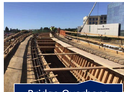
Bridge Overhang Construction
