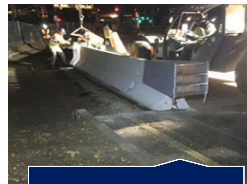
Installation of K-Rail
