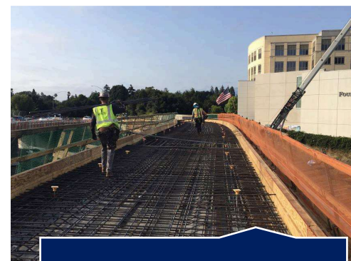
Rebar Placement
