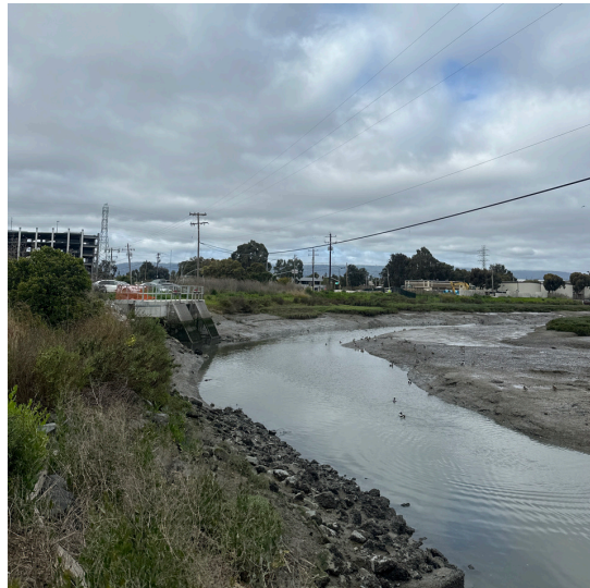
View C: Existing stormwater outfall at Flood Slough from Marsh Road within Bedwell Bayfront Park facing southwest.
