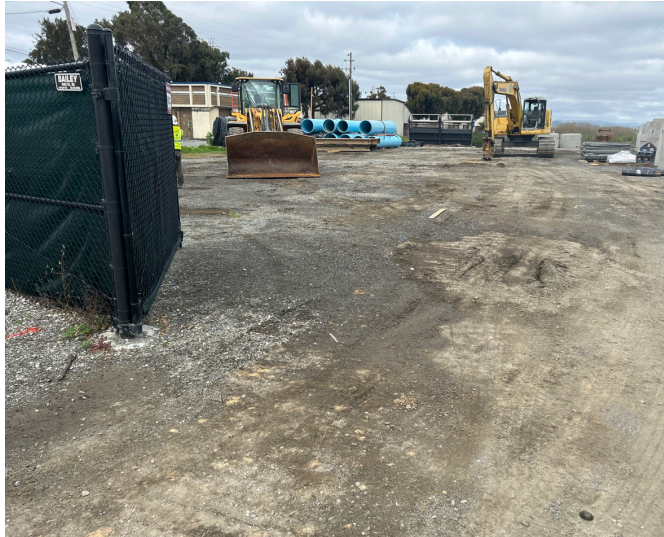
View A: Existing construction staging area within Bedwell Bayfront Park from Marsh Road north of park entrance.
