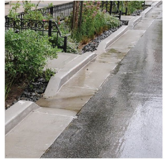
NEW CURB & GUTTER
