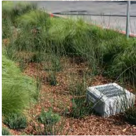
NEW DRAINAGE INLETS
