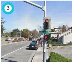
Bay St and University St: 9" signals reduce visibility of signal heads compared to 12" LED signals
