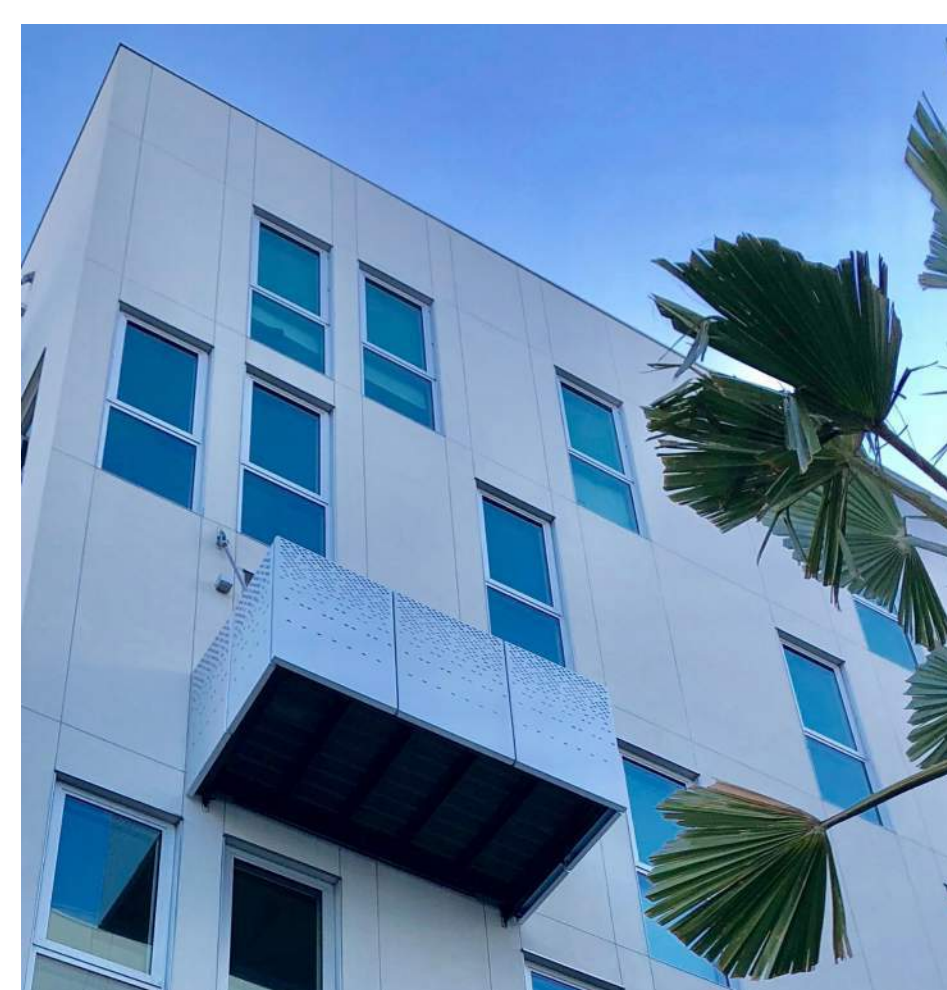
10 - Balconies with Perforated Metal Guardrails
