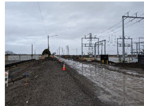
Bay Road Phase II Improvements
