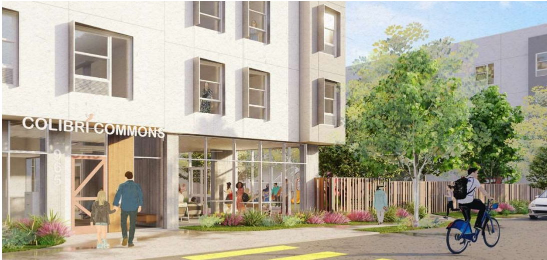
Affordable Housing Under Construction at 965 Weeks Street
