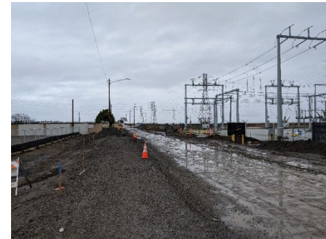
Bay Road Phase II Improvements
