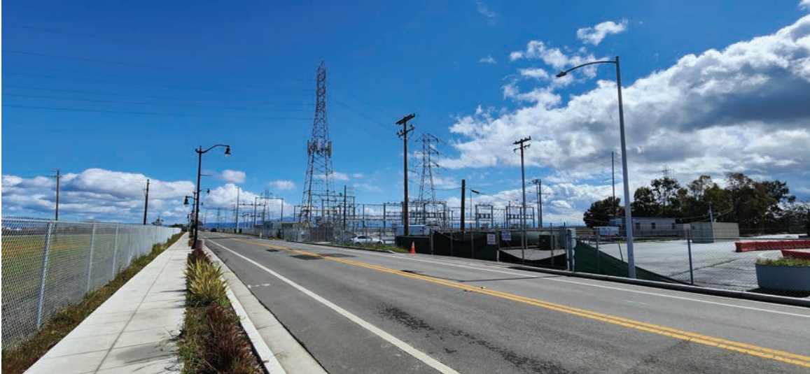
Photo 11: Industrial/warehouses, vacant lots, and transformers on Bay Road looking east towards the San Francisco Bay.
