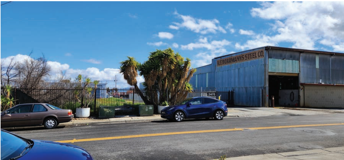
Photo 4: R.E. Borrmann's Steel Company building looking east on Pulgas Avenue.
