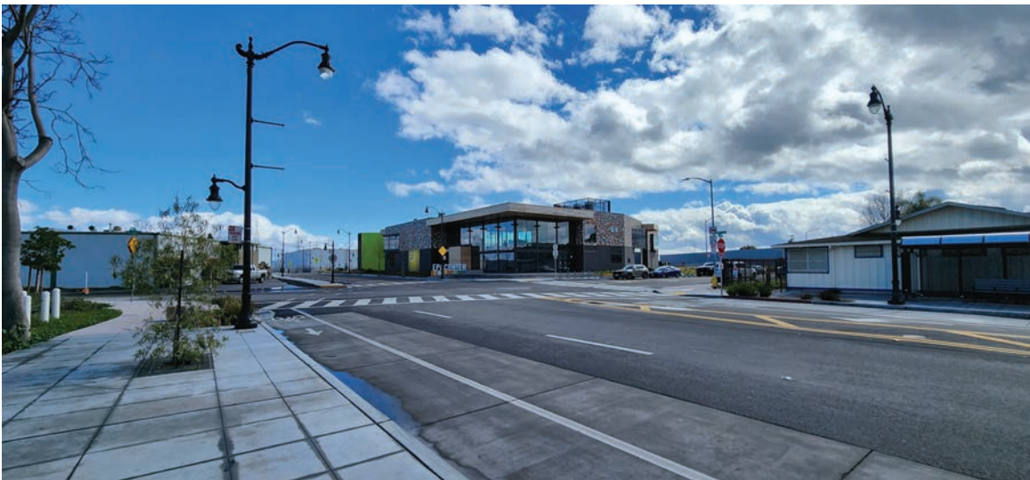
Photo 10: View of warehouses and the EPA Center looking west on Bay Road.
