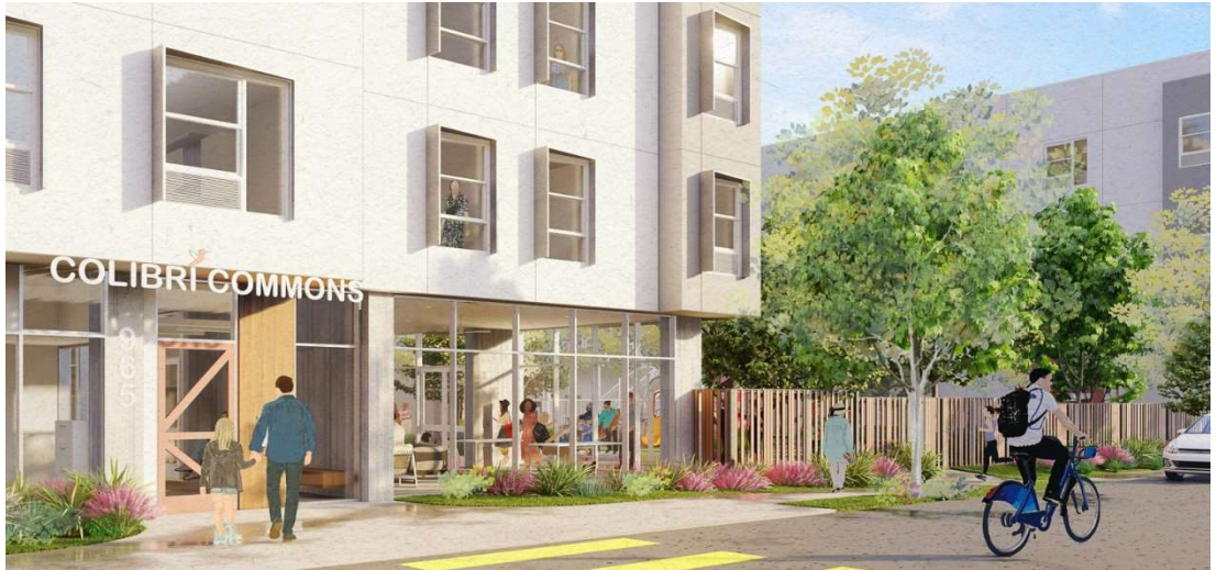
Affordable Housing Under Construction at 965 Weeks Street
